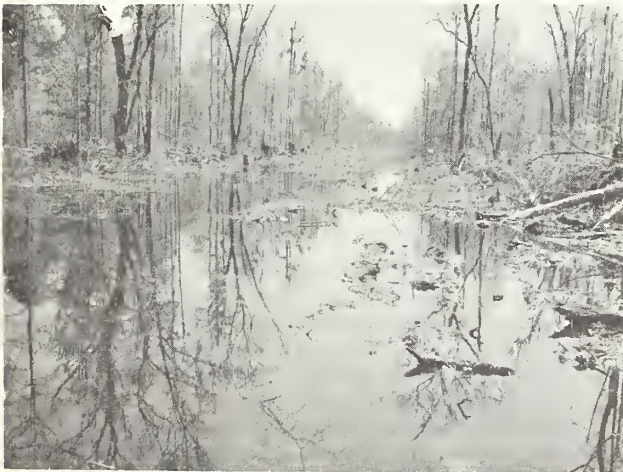
Right-of-way clearing for Main Drainage Canal.
